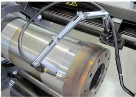
External Overlay welding
